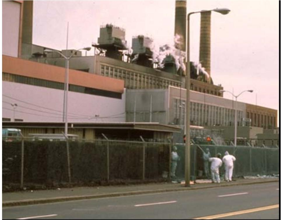
Painting crew at a major New England power station applies Endcor 4930 Series urethane primer-maintenance coating from Dampney Company Inc. to protect and improve the appearance of perimeter fencing. A single coat of the flexible, impact-resistant coating protects even marginally prepared rusted surfaces from corrosive salt air and industrial environments. Endcor 4930 cures under highly humid conditions in temperatures as low as 10°F (12°C).
